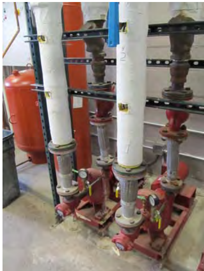
Mechanical system upgrades also included the installation of two new base-mounted circulating pumps
