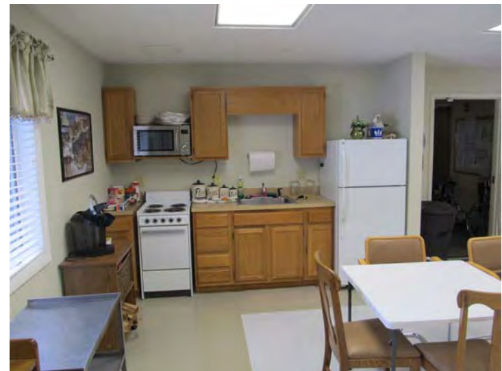
Kitchen area of community room lacks knee clearance under sink and a thirty-inch wide work surface with knee clearance underneath
