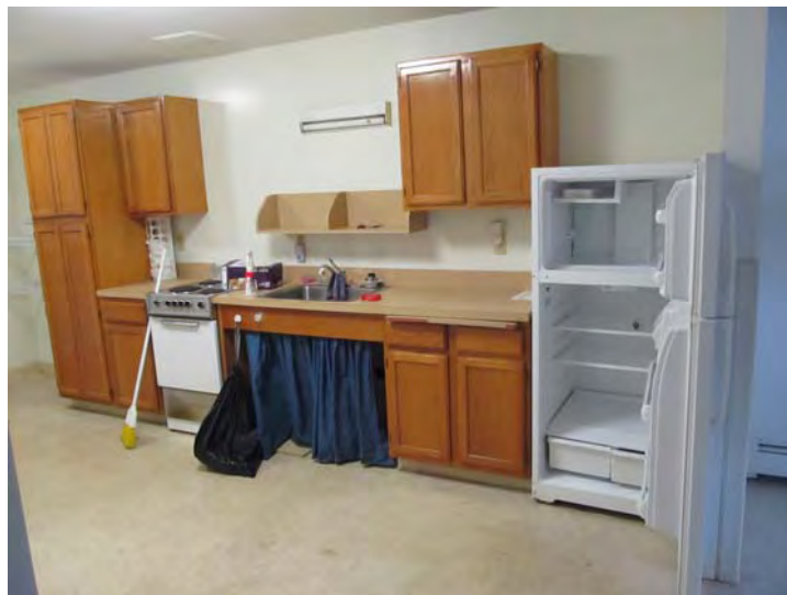
Handicap accessible unit kitchens include knee clearance under the sink but lack a thirty-inch wide work surface with knee clearance space
