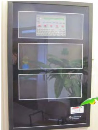
Fire alarm system serving the building has been upgraded in recent years and includes a fully addressable main control panel
