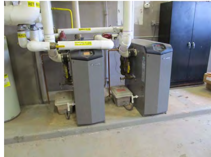
Recently installed boiler heating and domestic hot water boiler plant features two, high-efficiency, gas-fired boilers
