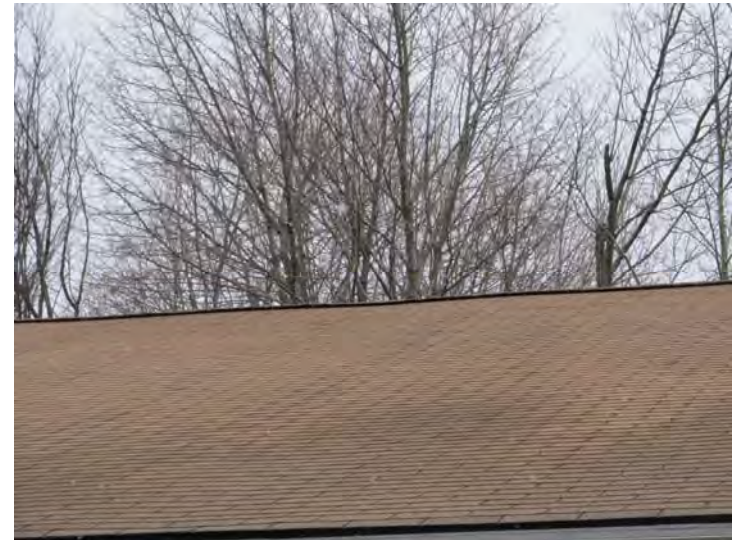
Three-tab roof shingles – No evidence of leaks observed or reported
