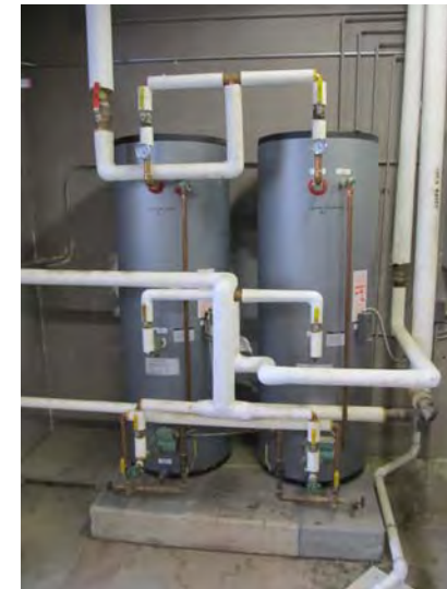
Indirect-fired domestic hot water storage tanks that work in concert with the boiler plant
